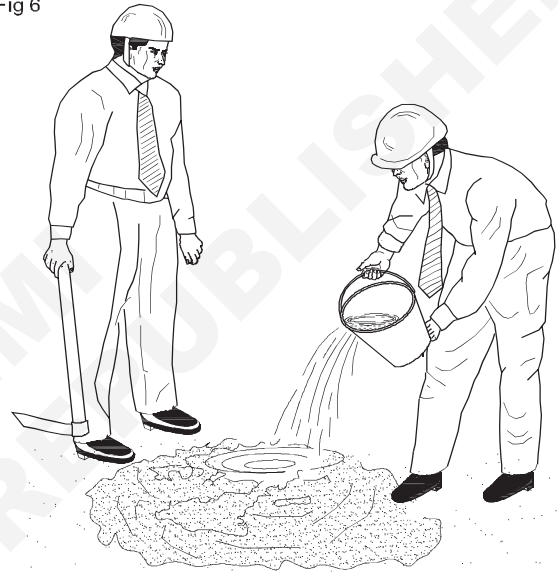
ADDING WATER IN DRY MIX
