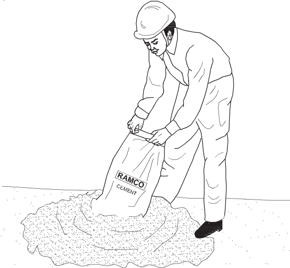
EMPTYING CEMENT BAG
